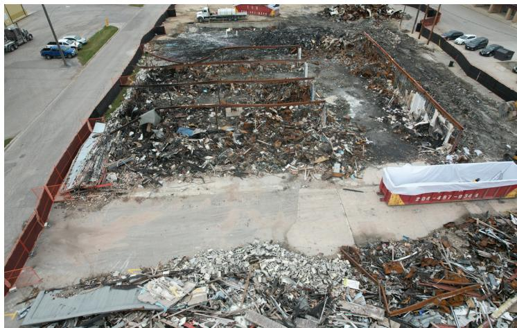
Among the most pressing concerns were the presence of asbestos-contaminated materials and hazardous runoff from fire-suppression efforts.
